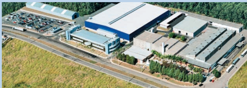
The new pump assembly hall with its state-of-the-art architecture measures 7200 m 2 .
