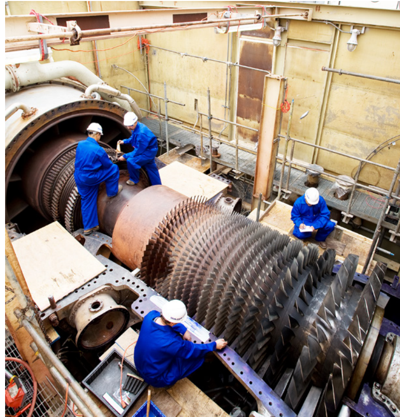
GE 7FA turbine onsite inspection
