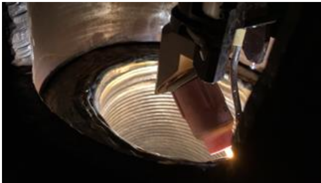
Picture 1: On site nozzle repair
